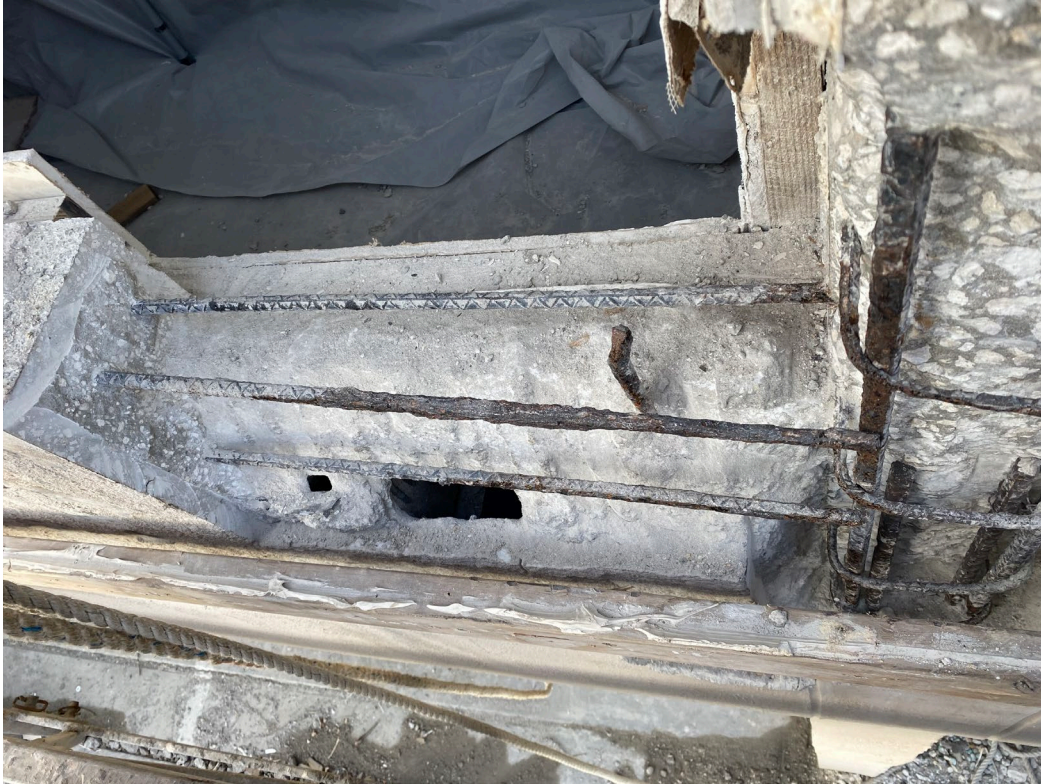
Picture 1: Unit 103 window sill repair
